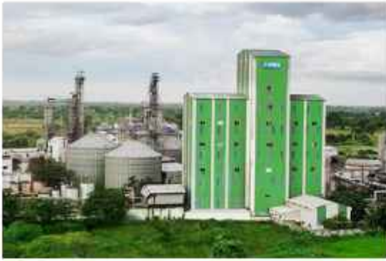
INDAMARA POULTRY FEED PLANT
